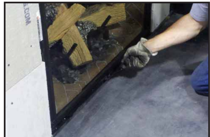
Figure 14.13. Securing Bottom Glass Clips
